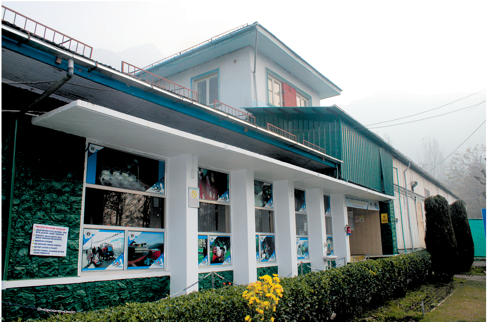
Milk processing plant in Cheshmashahi, Srinagar.
